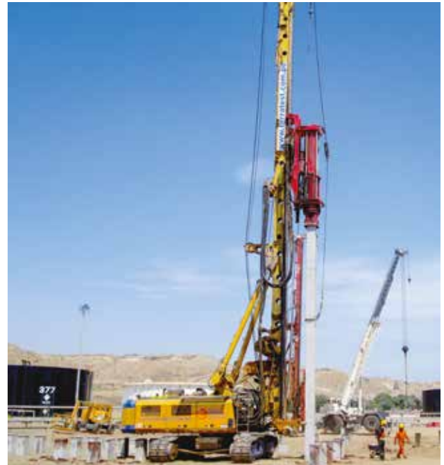
PILES IN THE TALARA REFINERY PROJECT – TALARA, PERU
