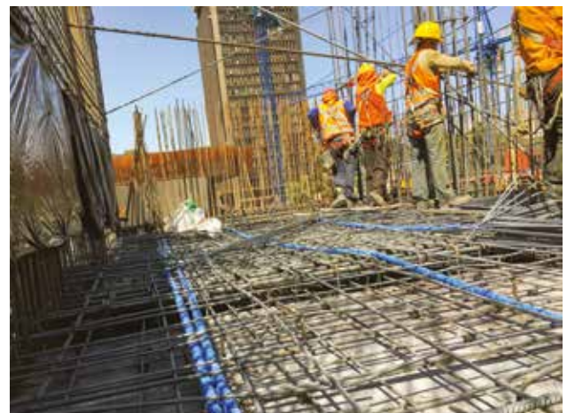
POST-TENSIONED SLABS IN STAGE 2 OF THE GABRIELA MISTRAL CULTURAL CENTER, SANTIAGO, CHILE
