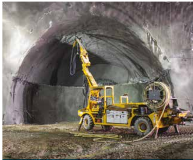
CIVIL WORKS FOR SHAFTS, GALLERIES AND TUNNELS IN SEGMENTS 2 AND 3, NORTH OF LINE 3 OF THE SANTIAGO SUBWAY SYSTEM, CHILE
