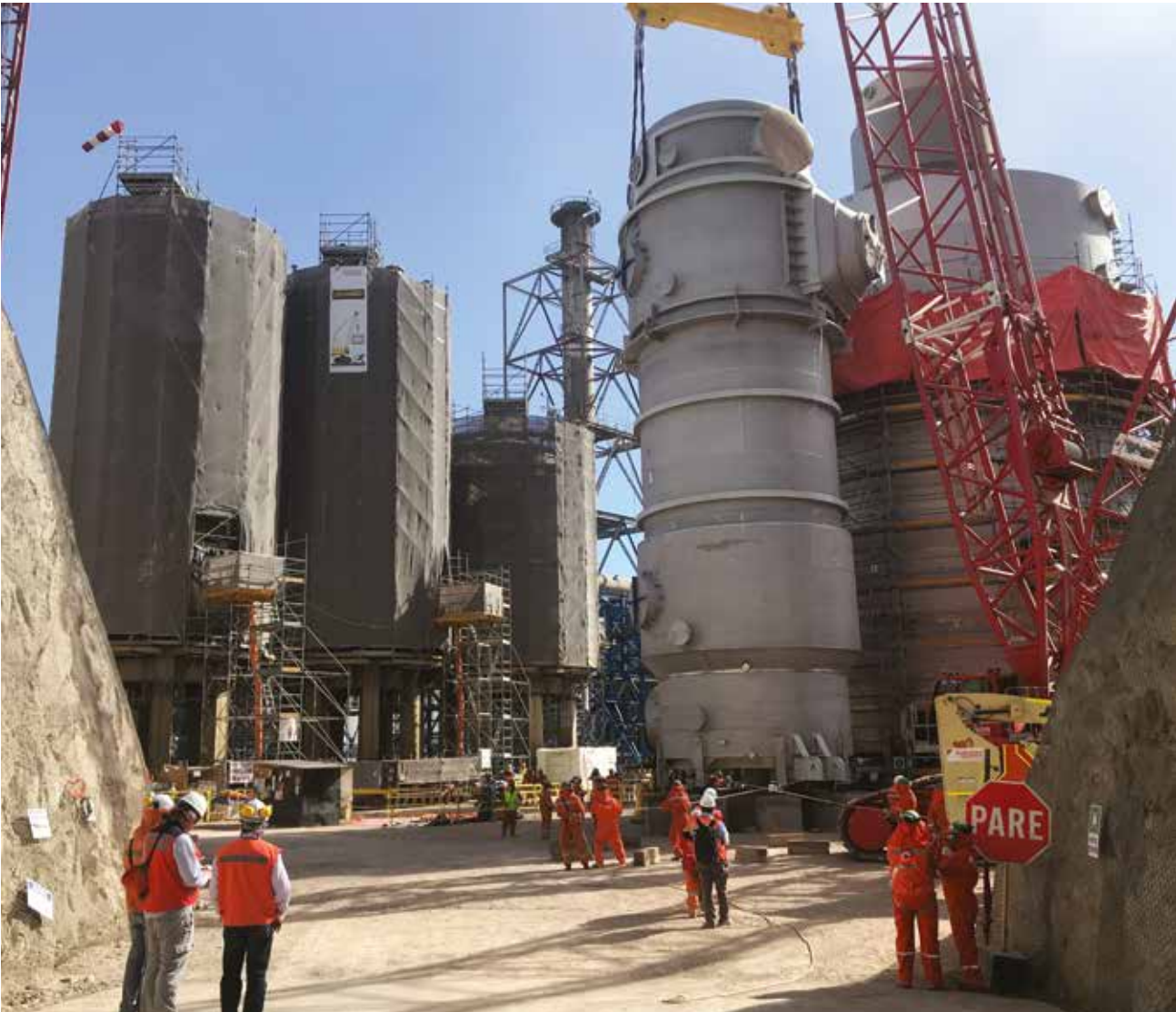
CIVIL WORKS AND ELECTROMECHANICAL INSTALLATION OF THE ACID 3 AND 4 PLANTS OF CODELCO, CHUCHICATAMA, CHILE
