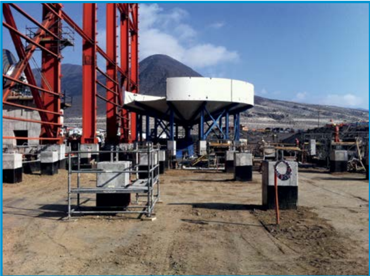
Hidroseparator, Planta Pellets, Huasco - Chile
