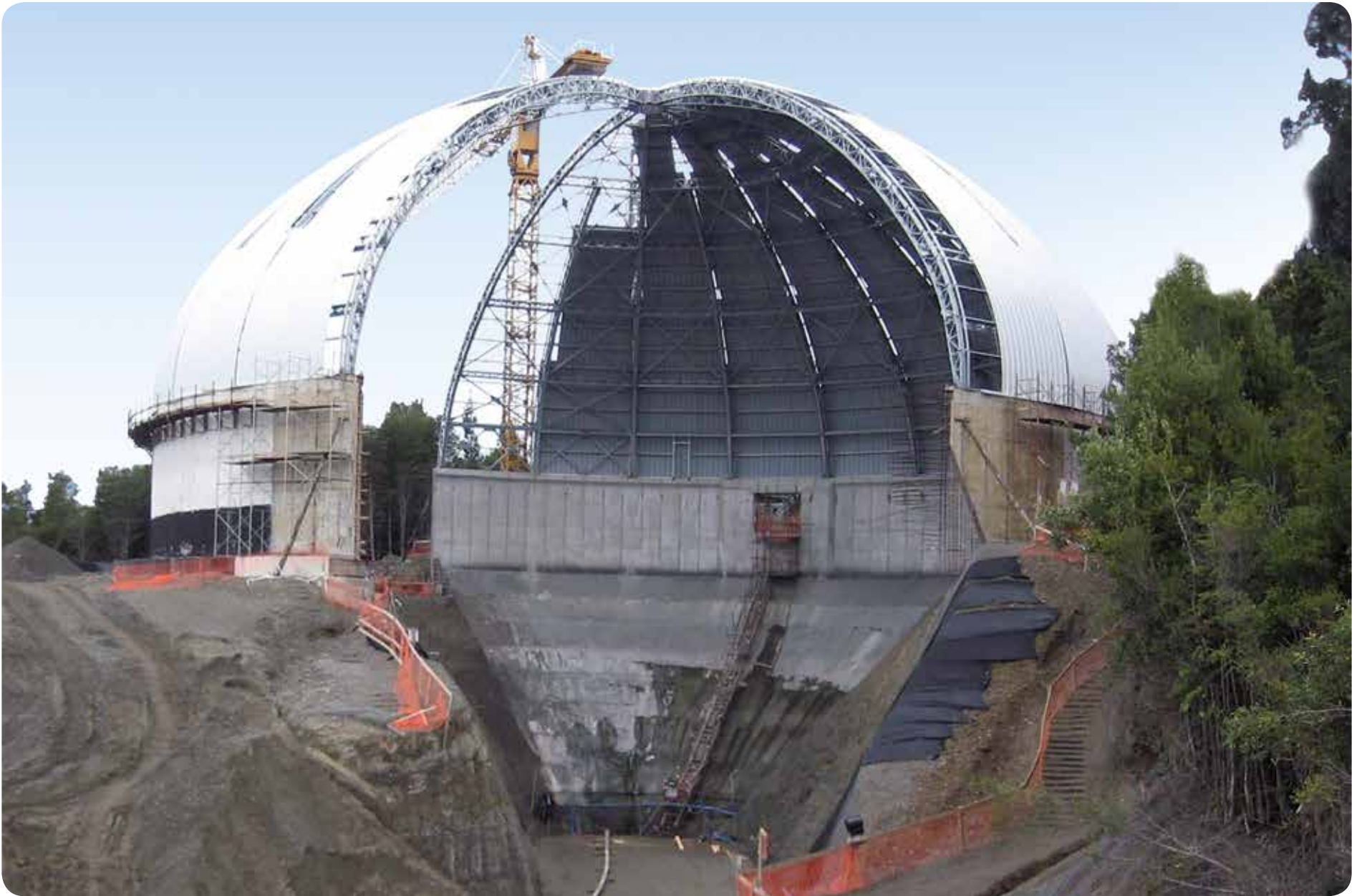
Domo puerto industrial Calbuco, Lafarge - Puerto Montt
