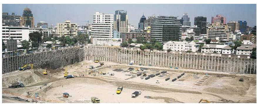
Post-tensioning anchorage - Costanera Center Mall
