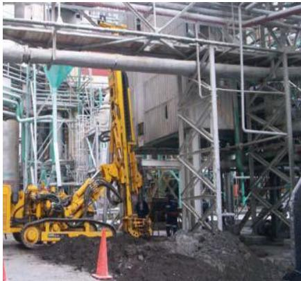
Micropiles drilling rig,
