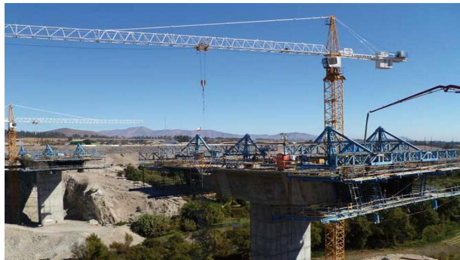
Balanced Cantilever Form Traveler Method, Huasco Bridge
