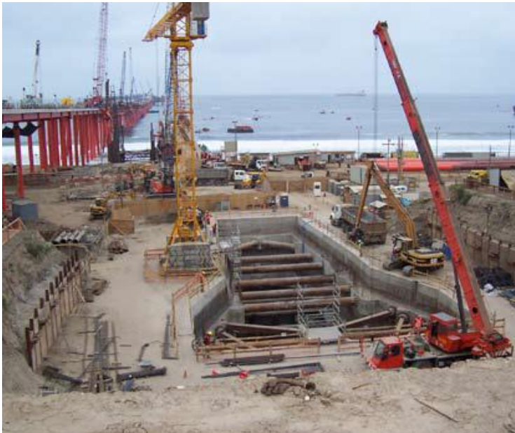
Muro Pantalla Sea Water Intake, GNL Quintero
