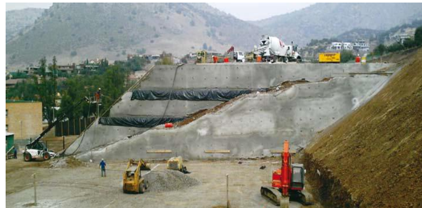
Soil Nailing, Colegio Everest
