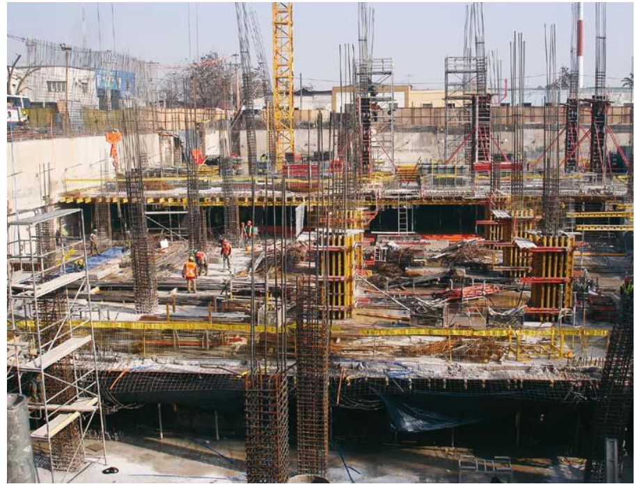
Losa Postensada Mall Plaza Alameda
