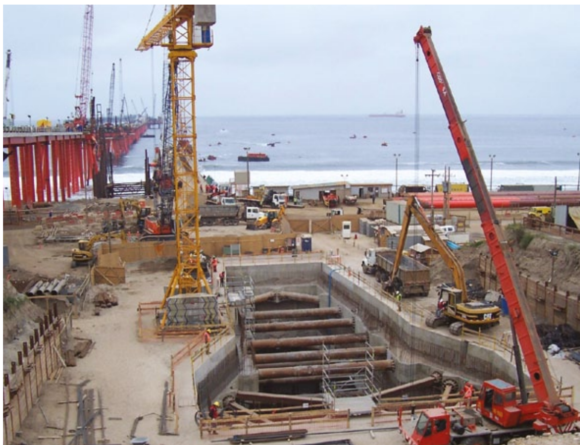
▀ Muro Pantalla Sea Water Intake, Terminal GNL Quintero
