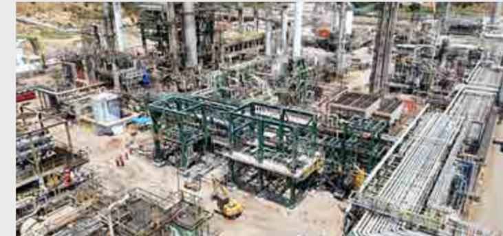
The project entails the construction and assembly of the sour water stripping (SWS) plant, the sulfur recovery plant (WSA) and associated connections to be done at the ENAP Aconcagua Refinery, located in the Region of Valparaiso. The purpose is to improve the reliability of sour water stripping and sulfur recovery to ensure the utilization rate at the Aconcagua Refinery. The scope of the work contracted by our customer, KT-Kinetics Technology/
