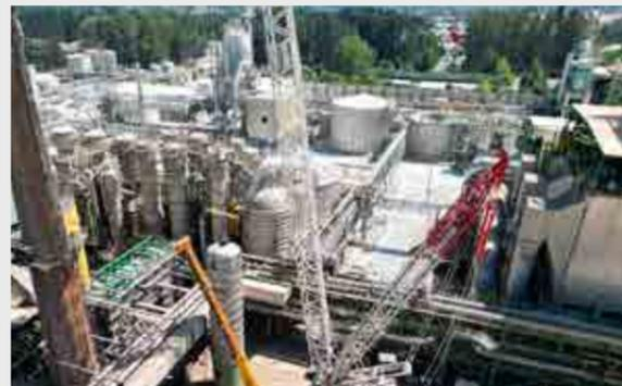
EIMISA finished the SF2 Evaporator Upgrade at CMPC'S Santa Fe Plant located in Nacimiento. This project encompassed the modernization of the Line 2 evaporator plant and included electromechanical assembly, pre-assembly, pre-commissioning and support during commissioning testing. The project was successfully concluded by the two-effect startup, an extraction column and methanol skid, together with the complementary equipment required for process optimization.
