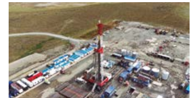
SERVICES AND INDUSTRIAL MAINTENANCE AT ENAP MAGALLANES
